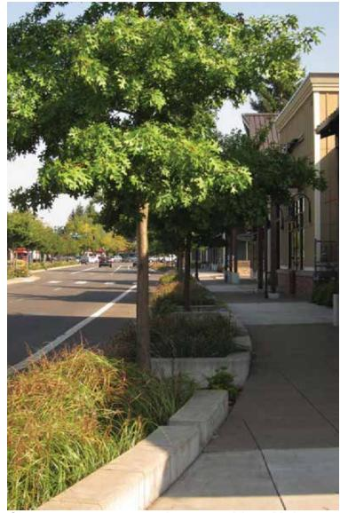
Stormwater treatment integrated into Main Street
