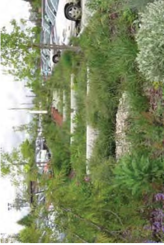
Parking Lot Rain Garden (Natural detention and filtration of parking lot rainwater)
