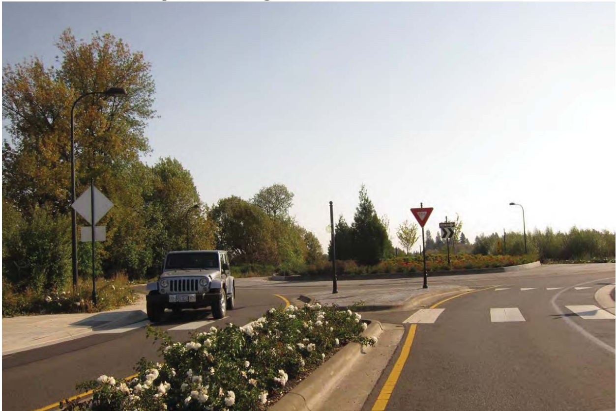
Pedestrian Refuge at Roundabout
