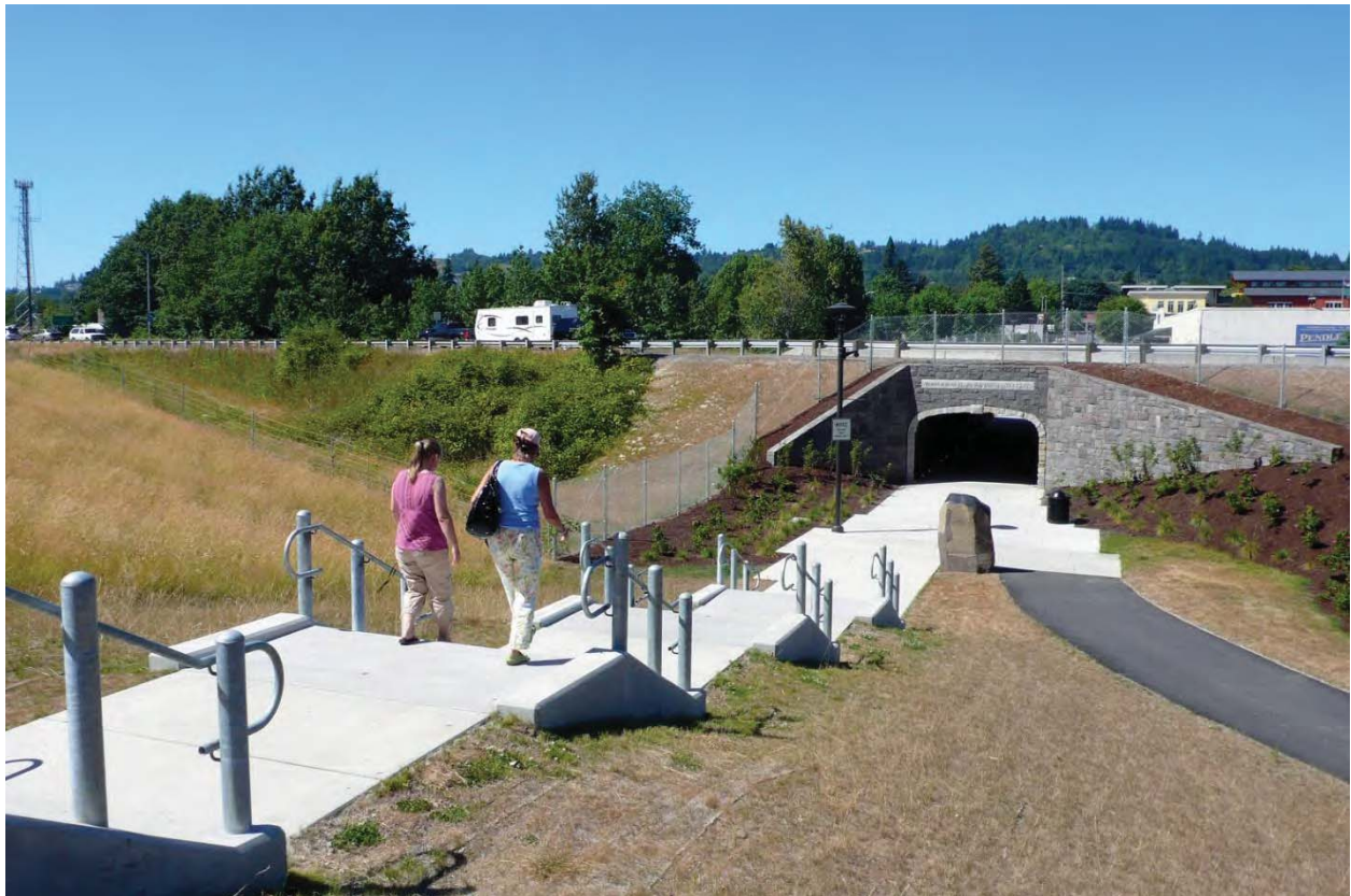
After: South end of SR 14 Pedestrian Tunnel, with stairs and ADA-accessible path connecting to fitness trail along the top of the Columbia River dike
