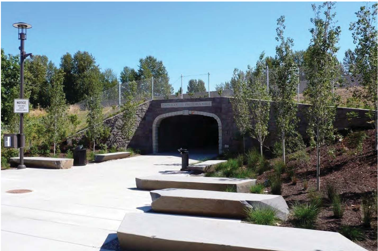
After: North end of SR 14 Pedestrian Tunnel, with pedestrian plaza
