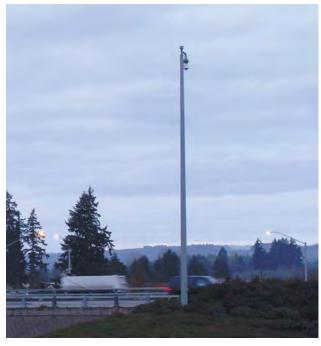
The CCTV camera mounted above the I-5/Wilsonville Road interchange provides a real-time video feed that allows ODOT to monitor and collect traffic information. The video feed is also available to all transportation users on ODOT's Trip Check website.
