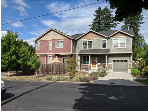
Two story duplexes with porches and front-facing garages
