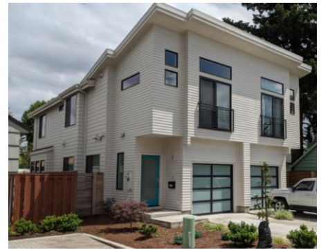
Four-pack quadplex of two-story attached homes; parking provided from two separate driveways
