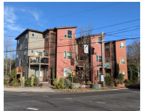
Triplex with shared surface parking located behind.
