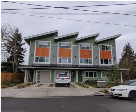
Attached quadplex with strong street presence; two homes with two parking and two homes with no parking.
