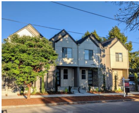
Quadplex built to front setback line; no parking.
