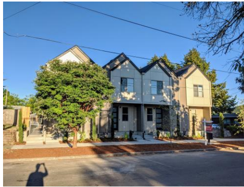
Pitched roofs and inset front patios create a small building effect; no parking in this example.
