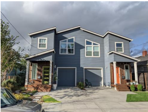
Garages and front doors on street-facing side at ground level
