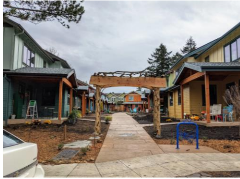
A prominent entryway features highlights the location of required walkways and circulation
